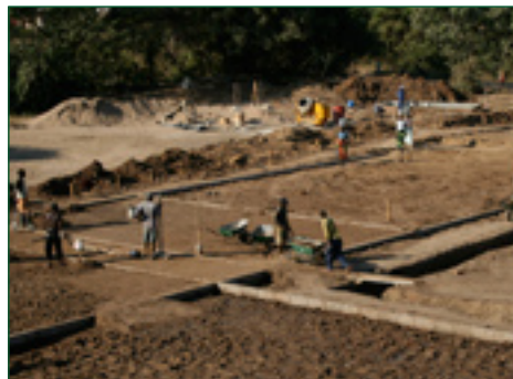
Construction of the new Lisungwi facility in June 2008
